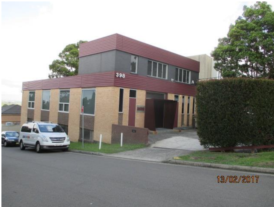
Photograph 5. Adjoining development to the south east.
