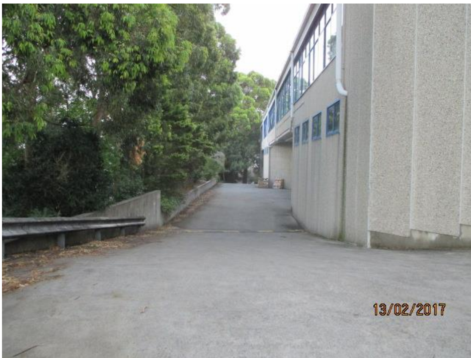
Photograph 3. Rear of the subject site demonstrating the elevated driveway and the vegetation on the adjoining sites.
