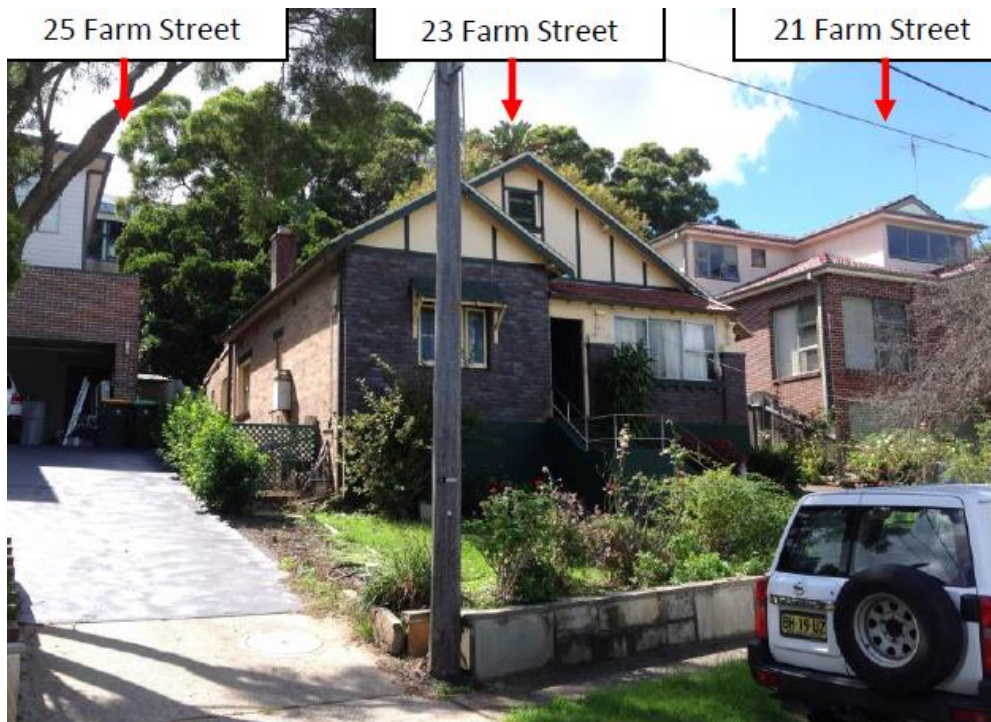
Photograph 8. 21 to 25 Farm Street.
